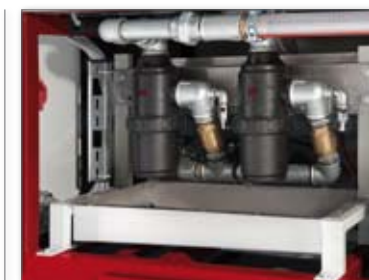
FILTER SYSTEM WITH BY PASS
